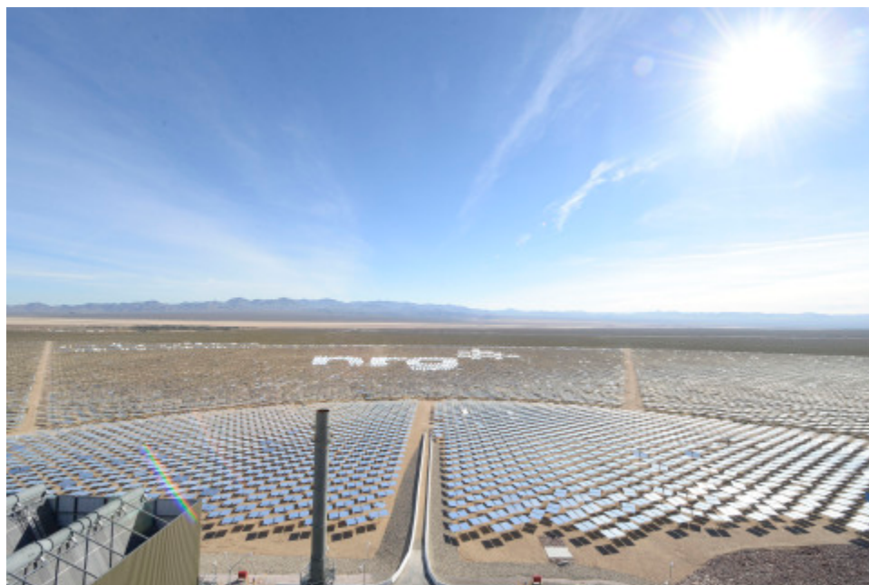
NRG Ivanpah Solar Electric Generating System (Photo: Business Wire)
