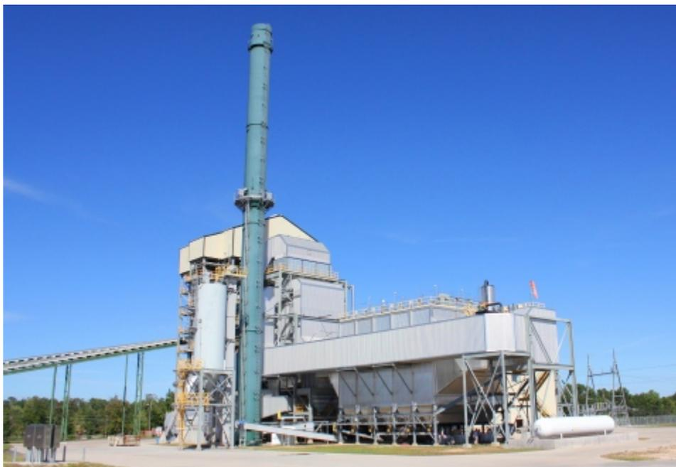
The Aspen power plant has the capacity to deliver approximately 50 MW to the grid and uses locally sourced clean wood-waste biomass as its fuel supply. The plant employs a stoker type boiler with particulate emissions abatement and has selective catalytic reduction for NOx control.
