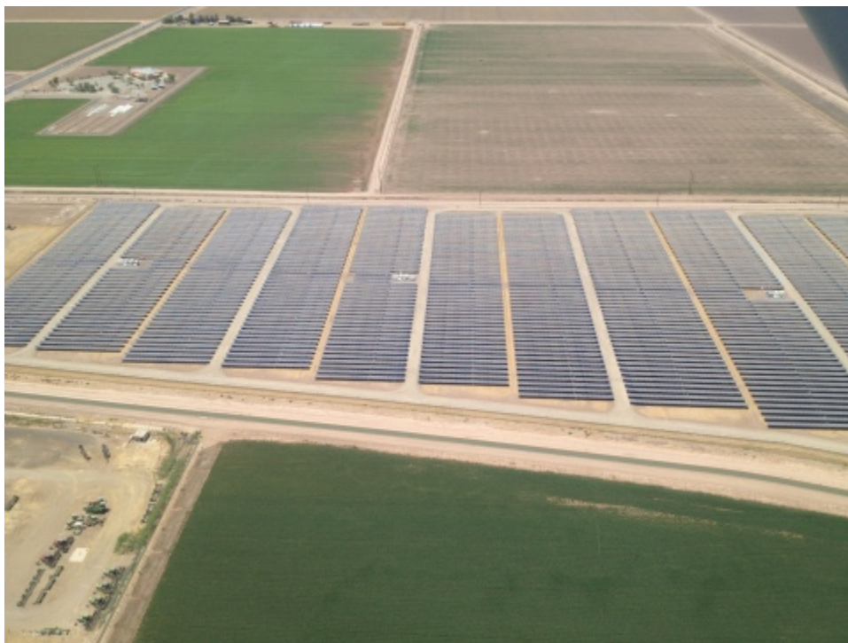
NRG Energy Community 1 Solar Facility (Photo: Business Wire)
