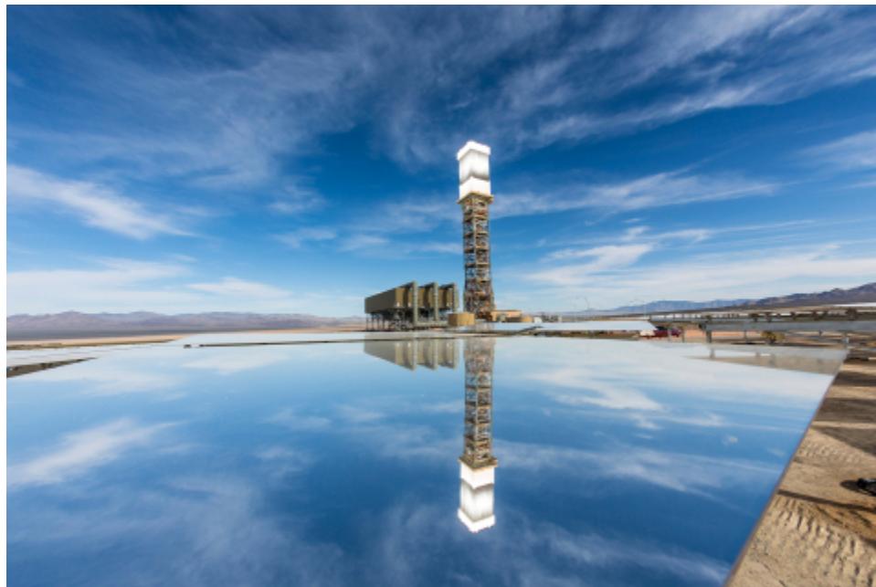
A view of the Ivanpah Solar Electric Generating System tower 1 and power block from the solar field. Each tower is 459 feet tall, 150 feet taller than the Statue of Liberty. (Photo: Business Wire)
